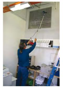
Commissioning return air: testing to ensure required air rate is being achieved (Source: AIRAH)
