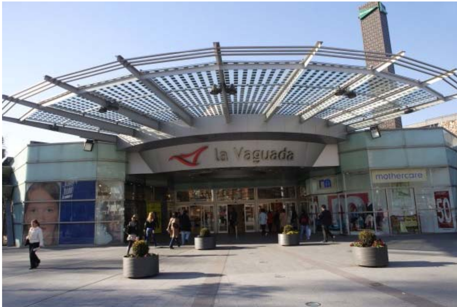
La-Vaguada entrance PV canopy 5.2kWp Madrid
