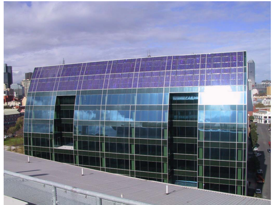
43kWp Melbourne University PV glazing façade, Australia
