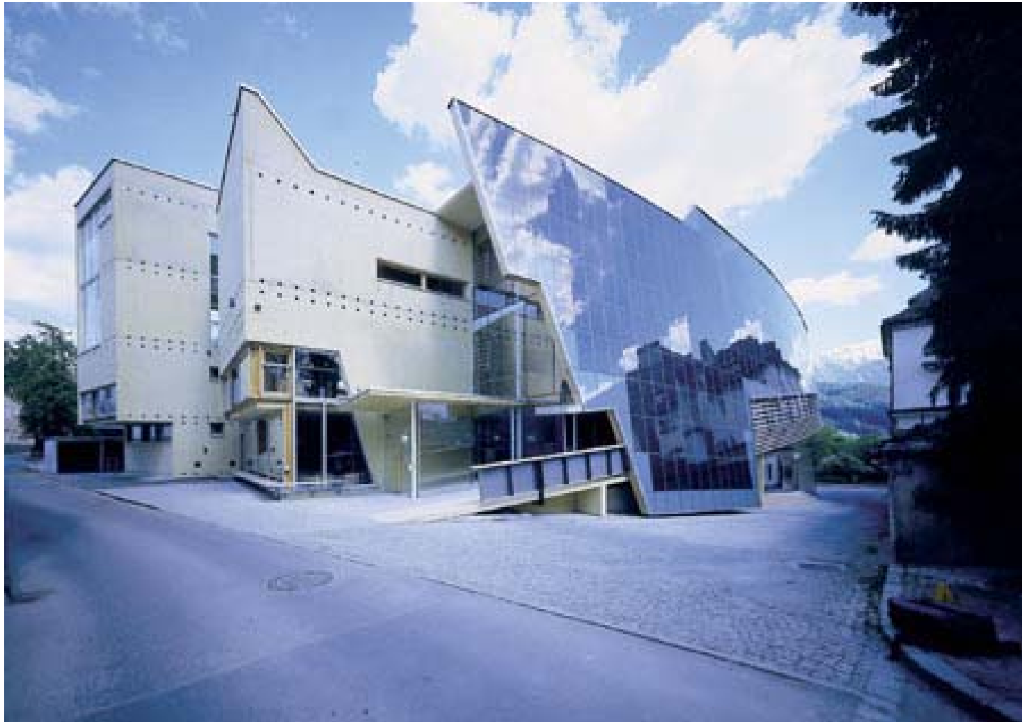
13 kWp PV at Vocational School Tyrol, Austria
