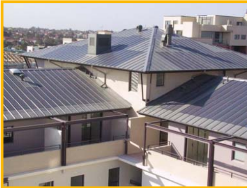
Kogarah SYDNEY 160 kWp
