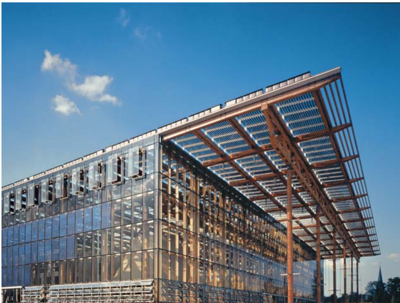
1MWp Mont-Cenis-Academy building, Herne Germany
