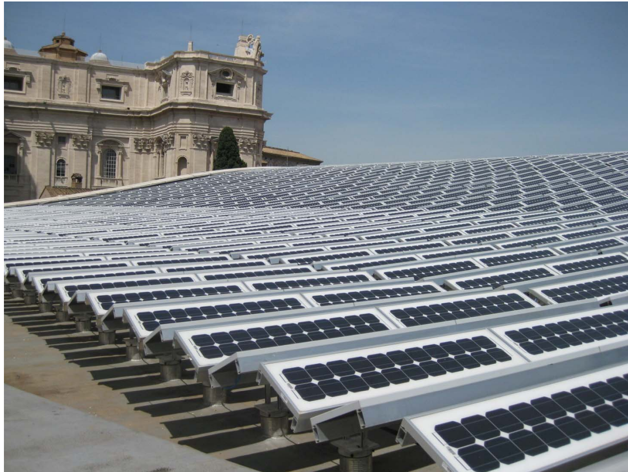
221kWp of blessed Vatican PV
