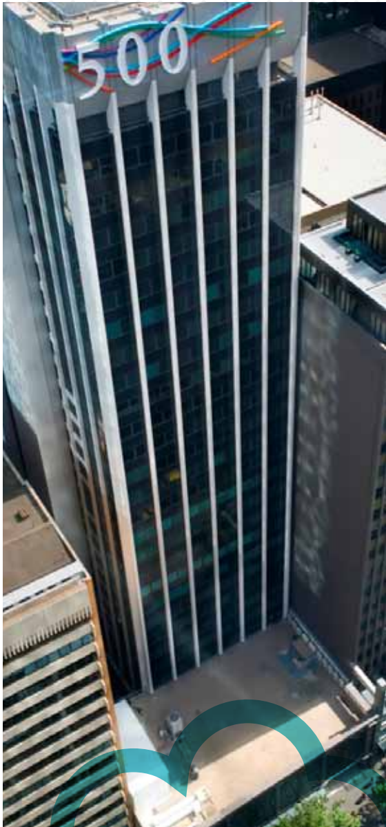
500 Collins Street - 5 Star Green Star - Office Design v1
