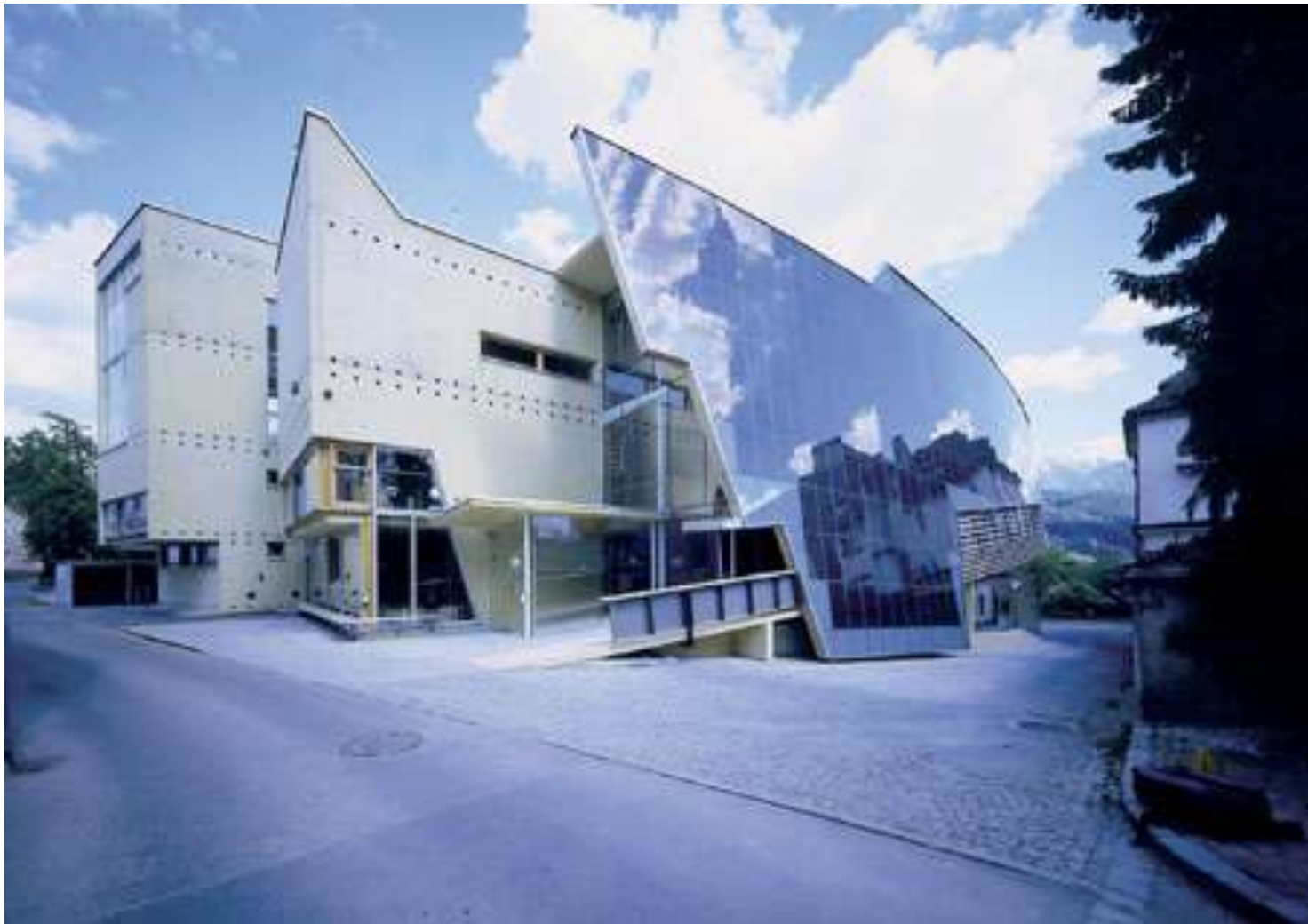
13 kWp PV at Vocational School Tyrol, Austria
