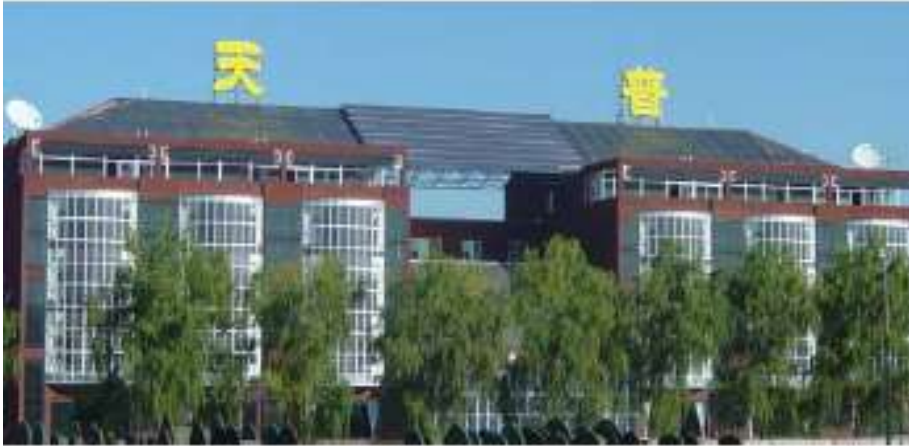
Tianpu, Beijing Grid-connected system (50kWp)
