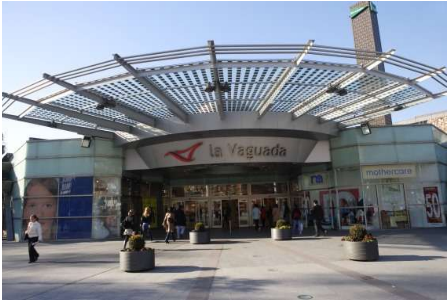
La-Vaguada entrance PV canopy 5.2kWp Madrid
