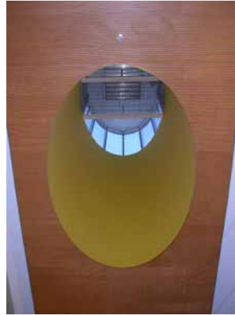
View up into solar chimney.
