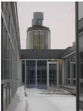
View through exterior courtyard of solar chimney beyond.
