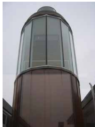
Close up of exterior detail of solar chimney.
