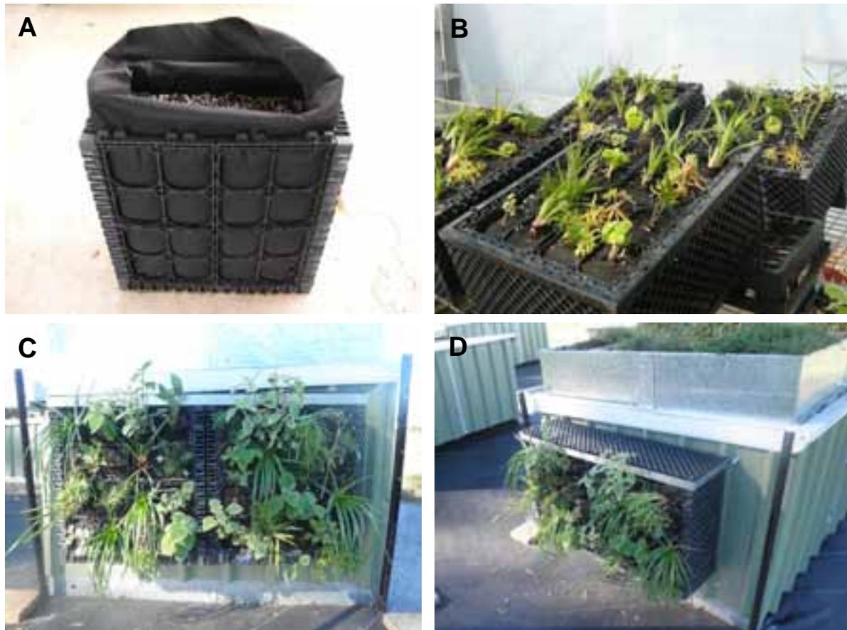
**Figure 10. Stages involved in the green wall installation**
