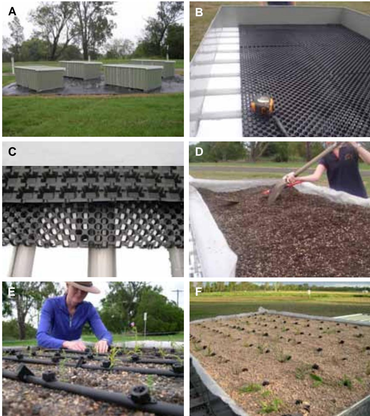
**Figure 2. Stages involved in the extensive green roof installation**
